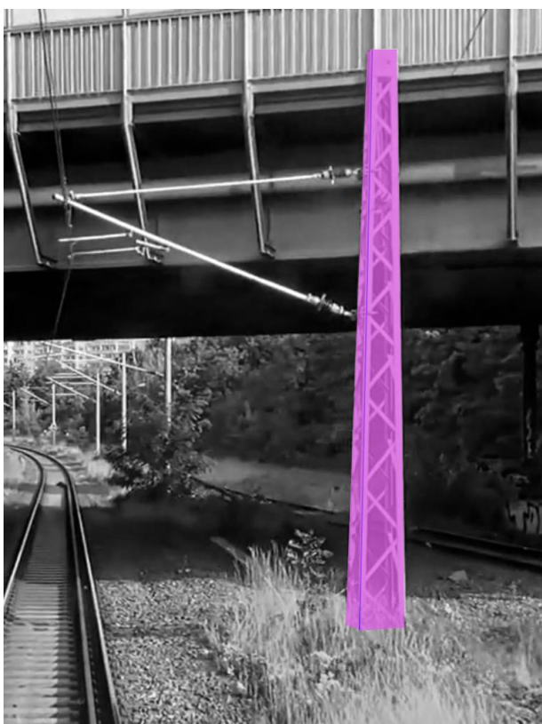
Correct annotation of a structured catenary pole (labelling ends on the blade of grass, i.e., foundation excluded)
