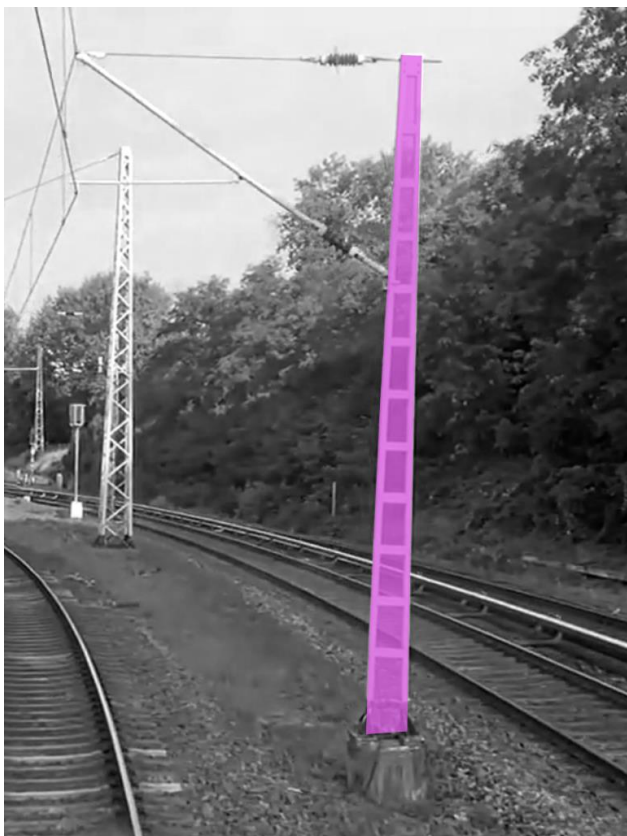
Correct annotation of a structured catenary pole (see the excluded foundation)
